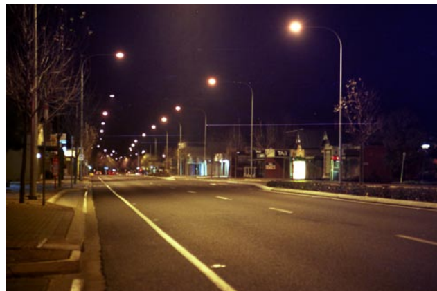
Quality full cut-off road lights on Sir Donald Bradman Drive reduce glare and facilitate night vision.
